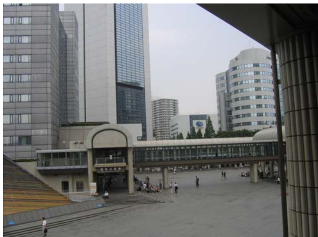
Fig. 1. View of the Kobe Convention Center.
